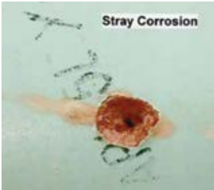
Fig. 3: Stray current corrosion of FBE coated steel pipe. This corrosion-induced failure is not related to blistering or shielding. The accelerated corrosion occurred in short time due to discharge of current at the defect holiday in the FBE coating.
