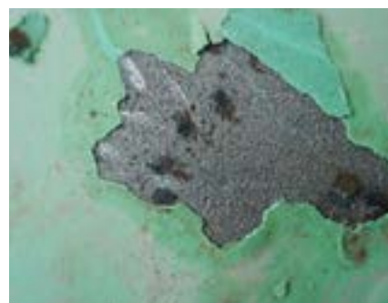
Fig. 2: Blistering of FBE coating on steel pipe.
